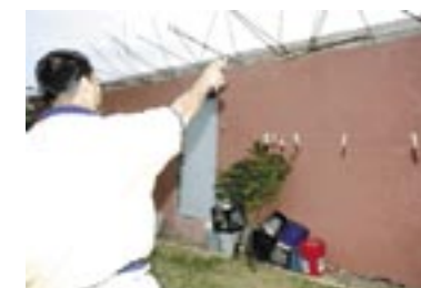
Rebar that will tie together future rooms.
